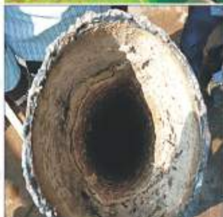
Before I.S.S Installation
