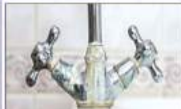
Taps are getting blocked and formed the white scales on the Taps
