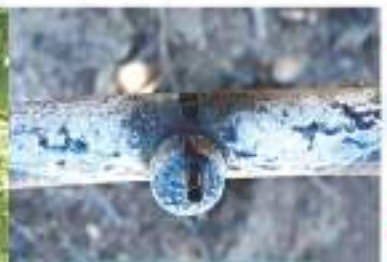
Drip Nozzle Before Converter
