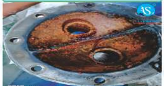
After installation At Heat Exchanger
