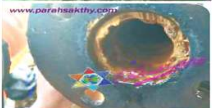
After installation At Cooling Tower
