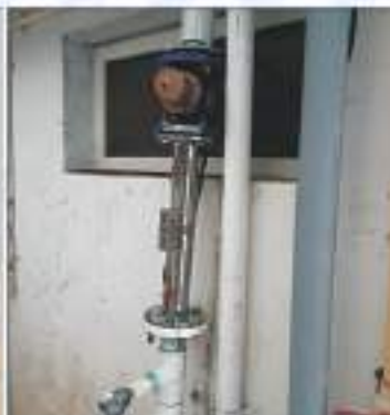
Reduce the flow of water due to formation of scales Due to scales formation the tiles loss their quality and shine
