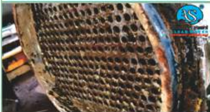
After installation At Heat Exchanger
