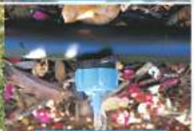
Drip Nozzle After Converter
